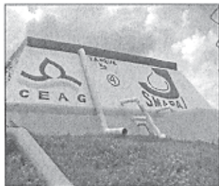
Tanque Superficial No. 4 Jaral
